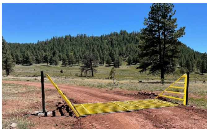
Figure 2. New cattleguards installed in 2023 to tie into the new Serna pasture fence.
